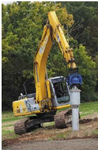
▲ Installing a screw foundation for a dual-axis tracking system (Deger-Traker) at Am Peterswald PV park in Germany: Bftec GmbH pre-drills the ground at the site and then the foundation is installed. The foundation's unusual form, which consists of a smooth side wall with a coil at the bottom (if necessary, two coils), guarantees a firm grip. The foundation can rotate in the ground without displacing or loosening the surrounding earth.
